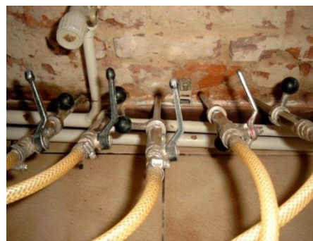
Figure 11 Chemical interruption Italy (Universita Ca'Foscari Venezia)
