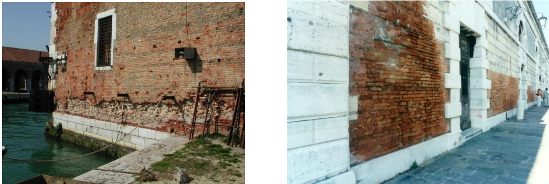
Figure 4 Alberaria Tower (Venice) and Salt emporium (Venice): horizontal courses of Istria stone blocks were used at the base of the walls to limit the capillary rise of water.
