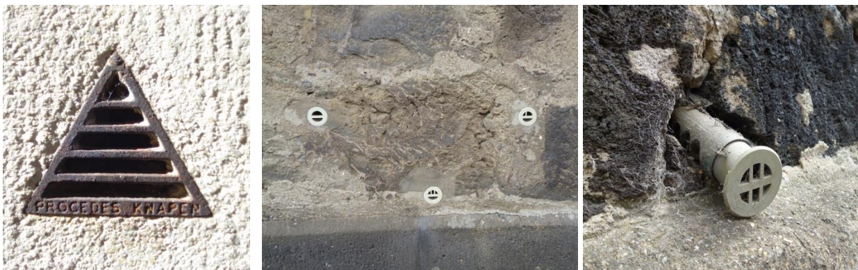
Figure 2, Different types of Knapen Siphons in a wall (Lubelli, B.)
