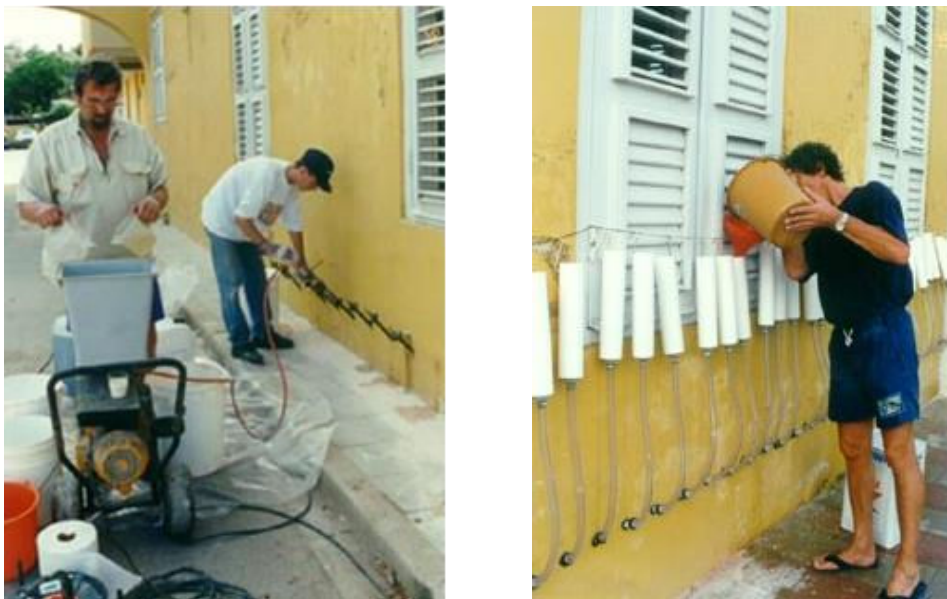
Figure 9 Treatment of a wall using pressure (injection)(on the left) and using only hydrostatic forces (impregnation) (on the right)[4]
