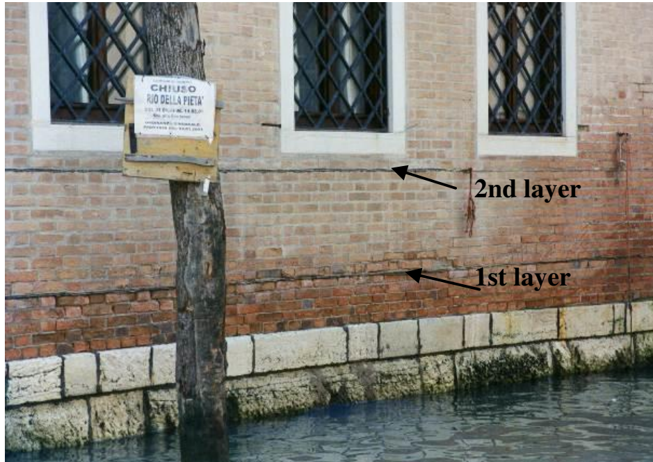
Figure 6 Presence of mechanical interruption (2 layers) in a building in Venice
